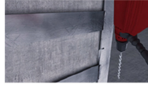
installing nozzles
